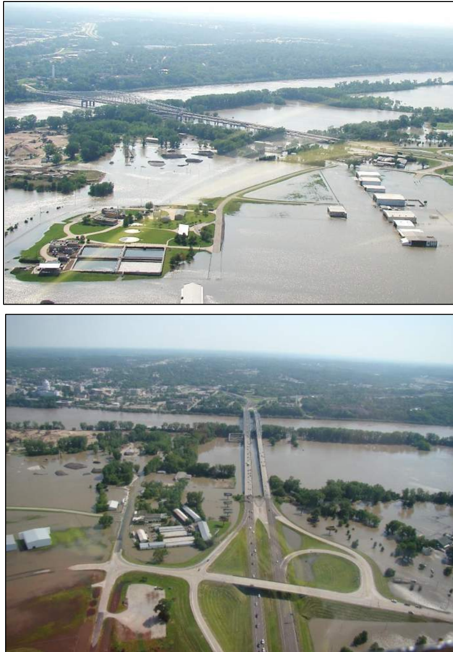
Figure 9. Missouri River Bridges (2019 Flood)
