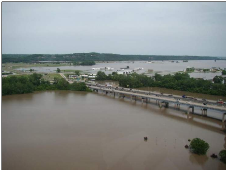
Figure 11. Capital View Levee from the Missouri River North of US-54 Bridge, Looking East – 2019 Flood
