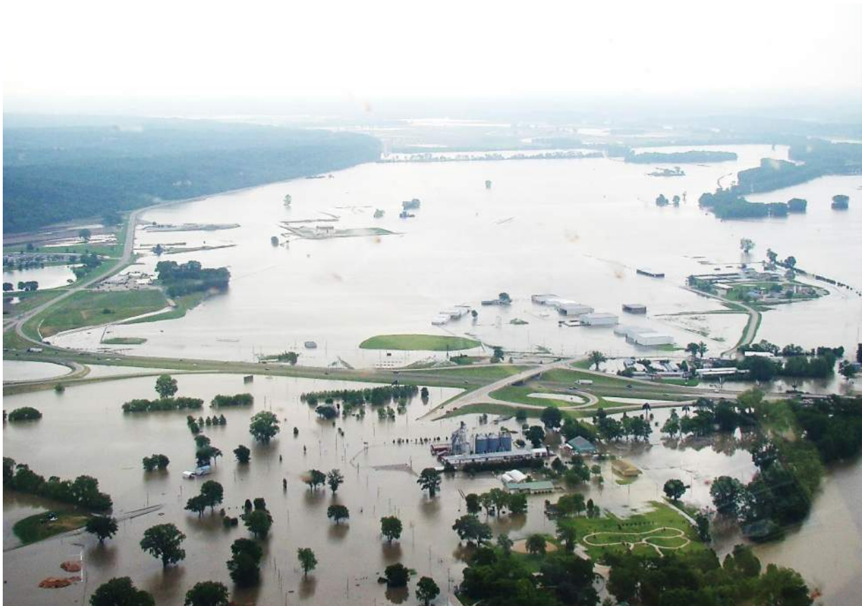
Capital View Drainage District, looking southeast toward inundated airport May 28, 2019
