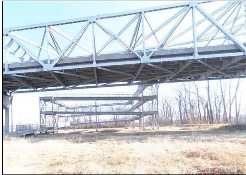
Figure 13. Pedestrian Access Ramp
